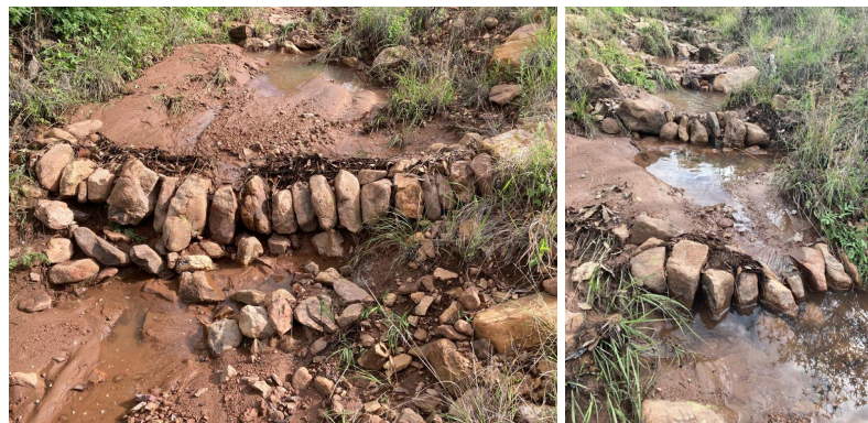
Examples of erosion control structures built by BRN following heavy rains.
